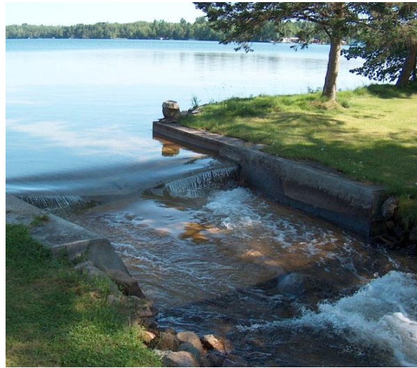
THE BIRCH LAKE OUTLET STRUCTURE COMPLETED JUNE 25, 2006
