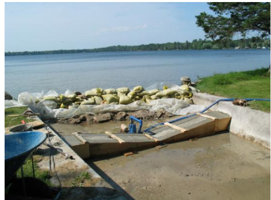
New Birch Lake "Dam" Under Construction June 23, 2005
