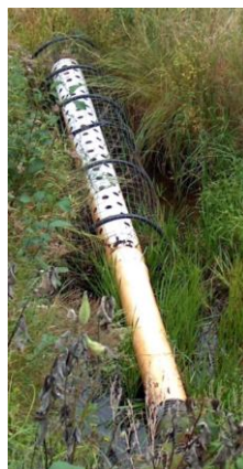
A Clemson Leveler: Typical Lake Level Control for Those Pesky Beavers
